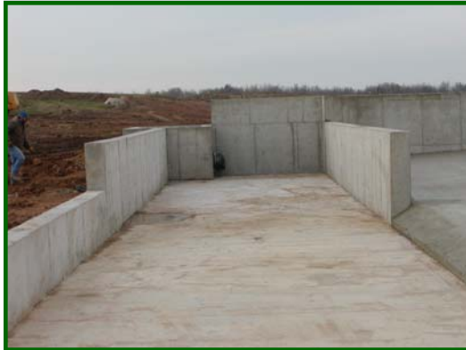
Sand Settling Lane
