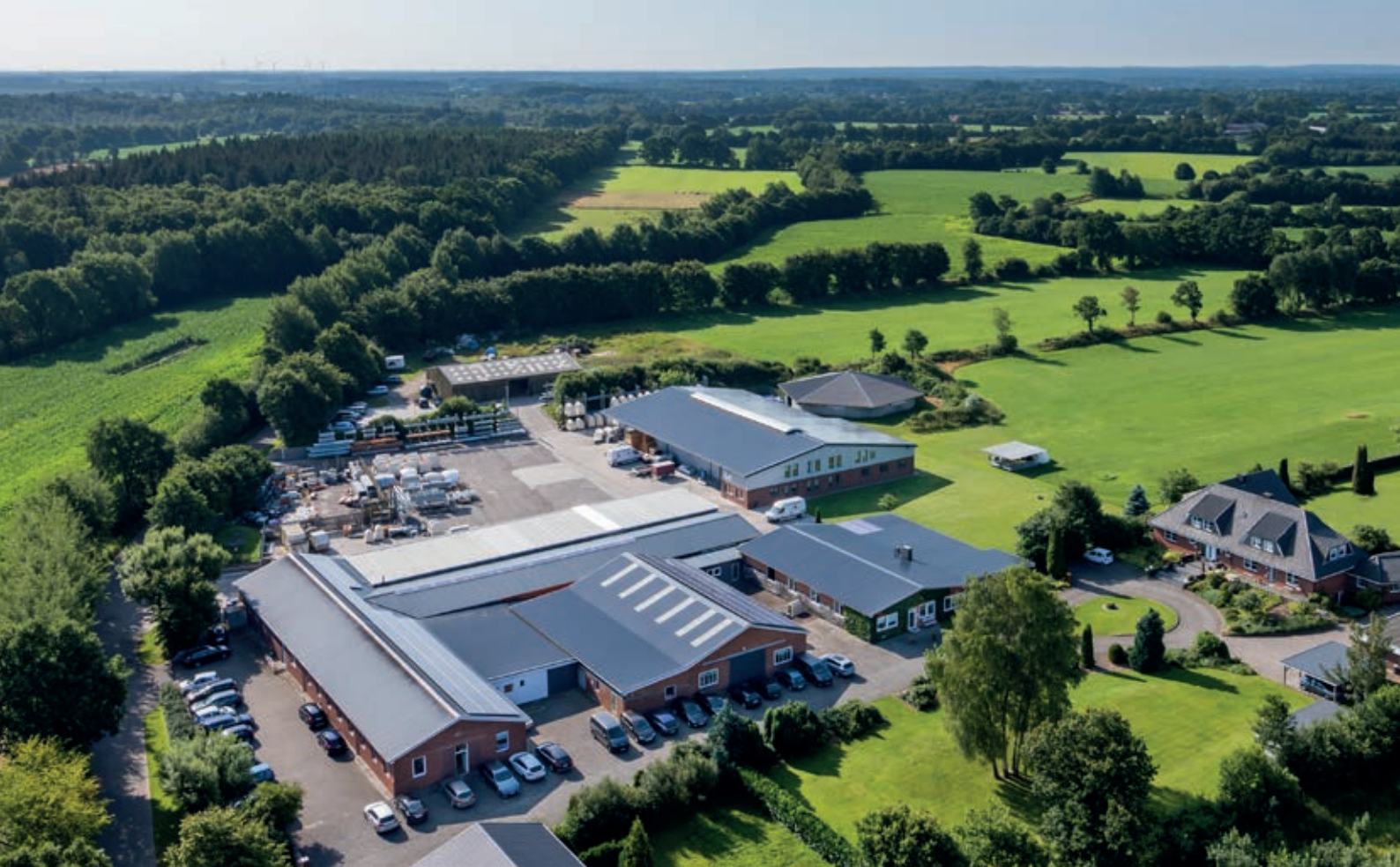
Holm & Laue company grounds in Westerröföfeld
