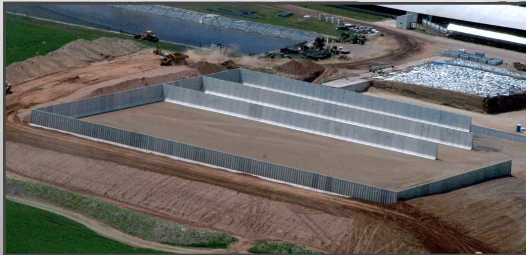
16' High Multiple Bay Bunker Silo Layout
